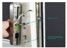
Apply marking take to both aites of the door and mark the position of the spindle. Above shows how the keyped will align on the door. The top and bottom bolts and cable position here are his constraint in
