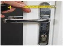
Miles the door closed, measure how the centre of the handle to the edge of the doorstop It rough be at least 0.82" to ensure the arount back will fit on the door.
