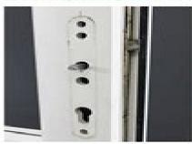
Open the stoor and remove the existing brandles and euro cylinder took. The euro cylinder is not required as the Stireline has a built in key over ride. 'Exerc the spindle in place.
