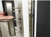
Office up the keypad to the door. Make sure that both stubs are aligned properly and tight. Locate the ignitide through the lock case. Feed the cable through the door cavity to the other side. Make sure the cubic does not bend hadk on basel.
