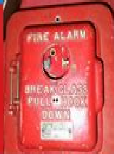
Vintage 1965 Simplex Type-4246-2 Fire Alarm Control
