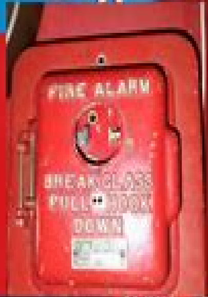
Vintage 1965 Simplex Type-4246-2 Fire Alarm Control
